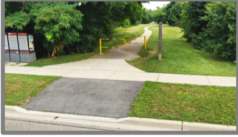
Gates, Fencing and Bollards
